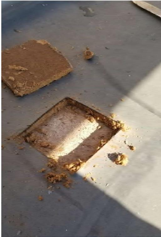
East Lower Roof (2<sup>nd</sup> Floor): rubber layer on wood core on concrete
