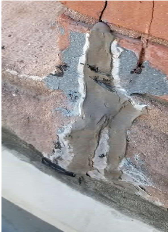
South Lower Roof (2<sup>nd</sup> Floor): **Asbestos-Containing** Black Glaze on Brick (Repair)( Presumed PCBs).
