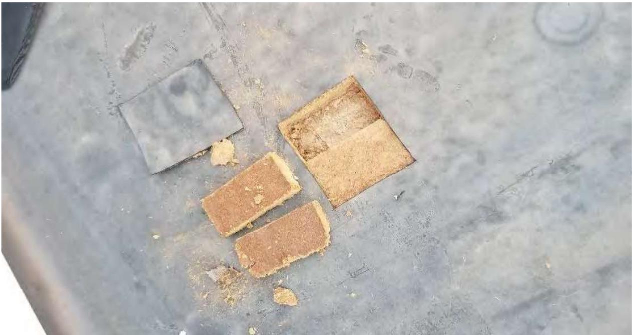
West Lower Roof (2<sup>nd</sup> Floor): Rubber on wood core on cement.
