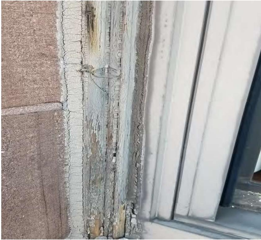
West Lower Roof (2<sup>nd</sup> Floor): **Asbestos-Containing** Brown Window Frame Glaze on Brick (Presumed PCBs)
