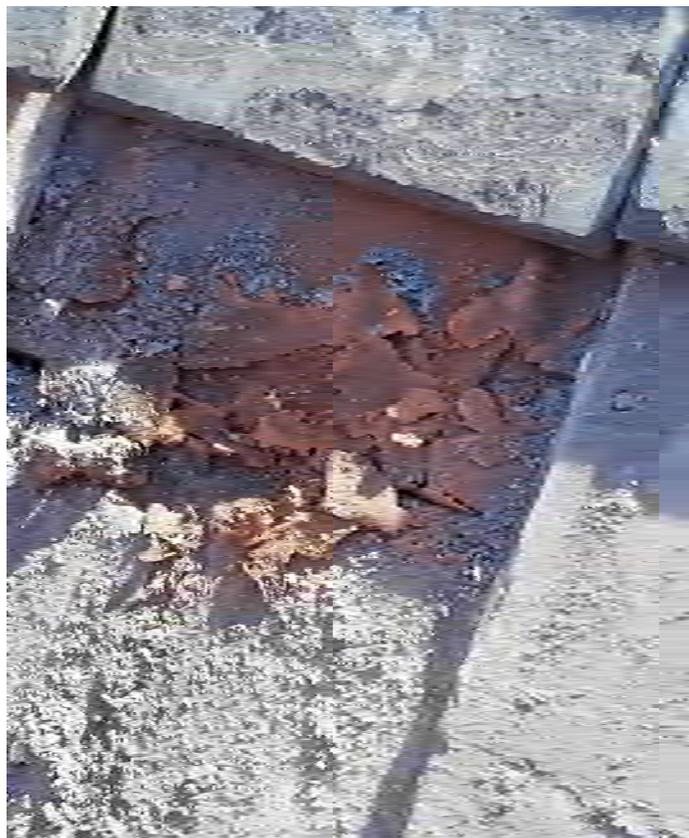
West Roof: Vapor Barrier Under Slate Shingle
