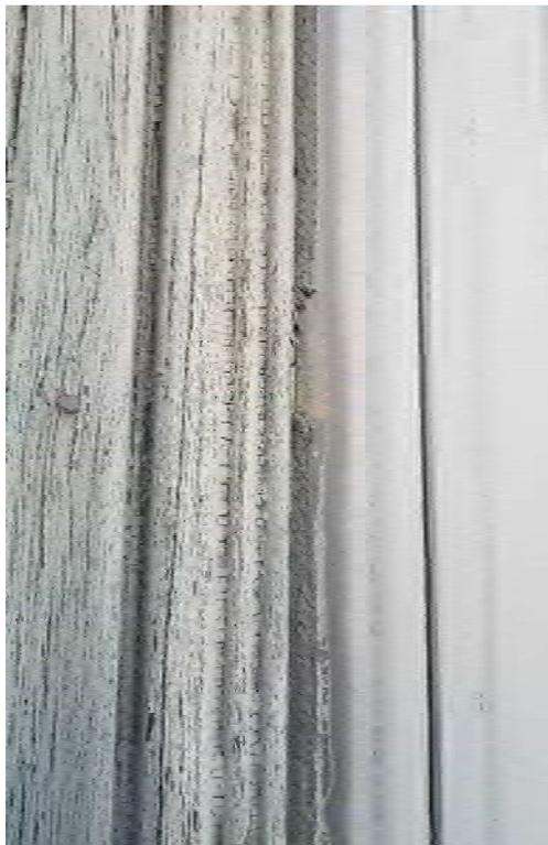
West Lower Roof (2<sup>nd</sup> Floor): **Asbestos-Containing** Brown Window Frame Sealant (Presumed PCBs)
