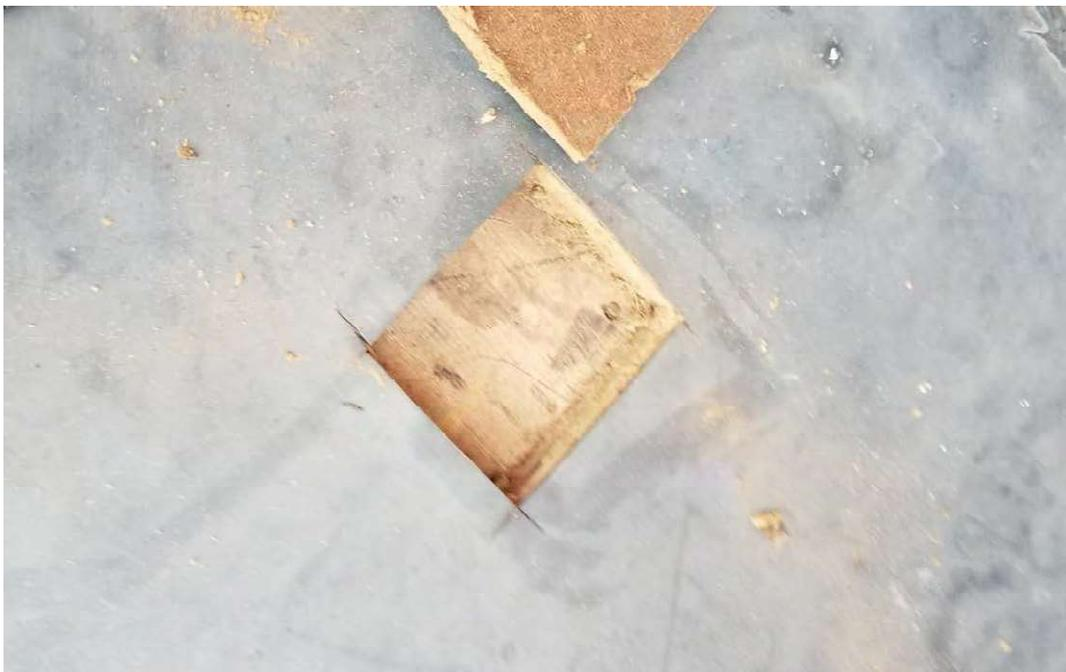
South Lower Roof (2<sup>nd</sup> Floor): Rubber on wood boards layered to make slope for water runoff.
