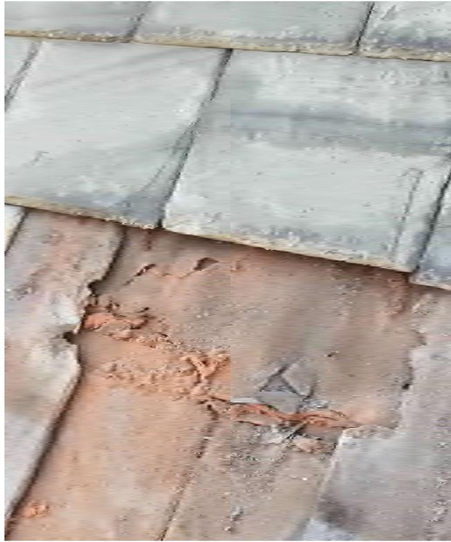
North Roof: Vapor Barrier under Slate Shingles.
