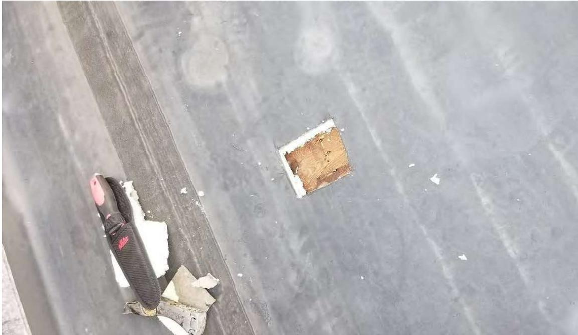
Center Roof: Rubber on Styrofoam Insulation.
